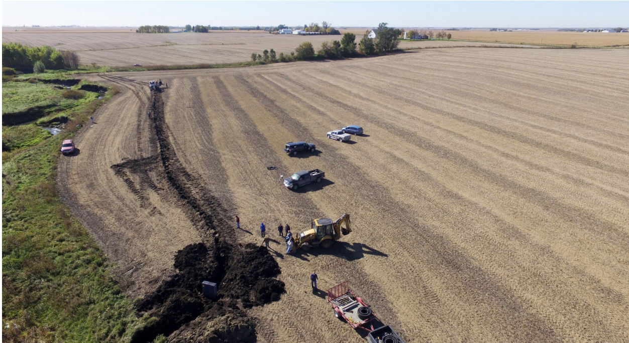
Saturated buffer installation in Story County, Iowa. NRCS/SWCS.
